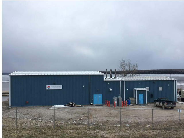
A new water plant built in 2019 was intended to end the boil water advisories in Eabametoong First Nation. But the community says the design is inadequate and relies on reverse osmosis systems. Photo by Michele Hakimian, resident of Eabametoong First Nation.
